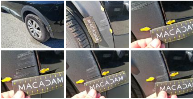
Bumper F, Deformed / Strained, Repair and paint (complete)
