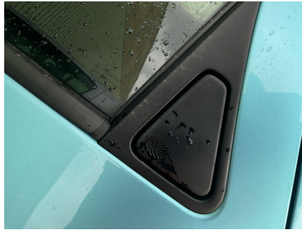
EXTERIOR - DRIVERS SIDE Handle Outer nsr; Scratched (Painted); UpTo 25mm Thru Paint
